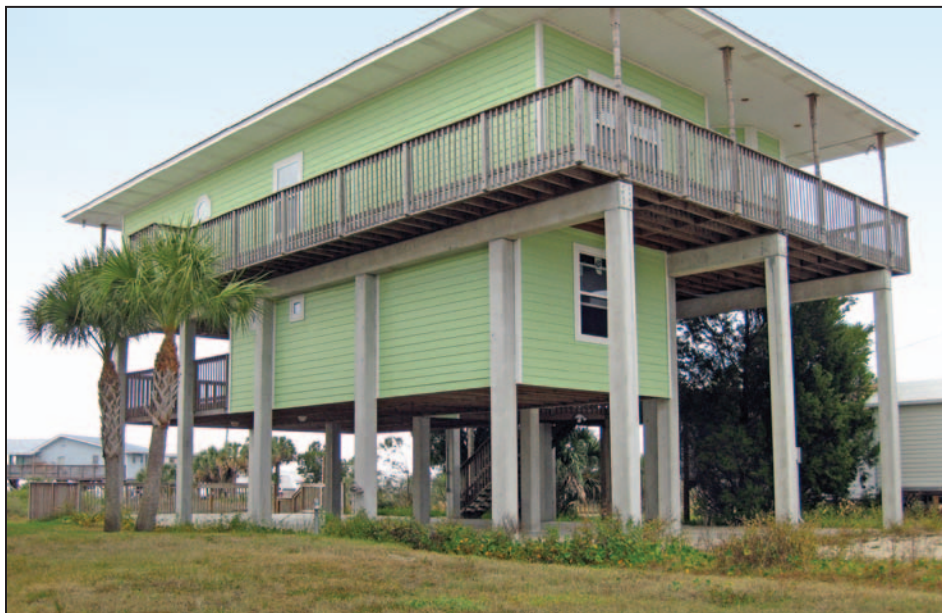
Figure 2-23. Above-grade enclosure (Perry, FL)
