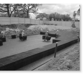
The R-Tank System includes five different module configurations, providing system height options from 2" to over 7' tall. And it delivers support for HS-20 and HS-25 traffic with cover depths from 6" all the way up to over 16'. Whether you're designing a project at the beach with minimal depth over the water table, or a deep system in the hills, R-Tank has you covered.
