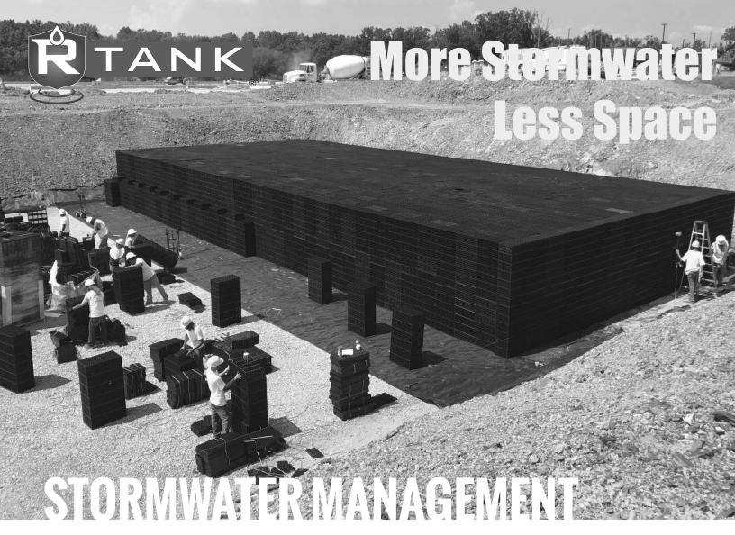
Is your stormwater detention system taking up too much space? Bring it down to size with the R-Tank System, the most efficient and versatile underground stormwater storage system available today. Whether you need to reduce your system footprint to resolve a utility conflict or free up space for a future expansion, R-Tank will give you the smallest footprint, provide more options for vehicular loading and cover depths, and deliver more installation versatility than any other system around.
