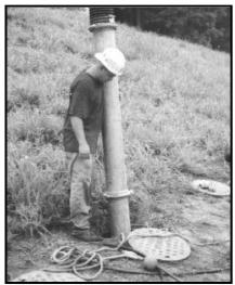
Vacuum truck quickly cleans the Aqua-Swirl<sup>®</sup> from a single chamber
