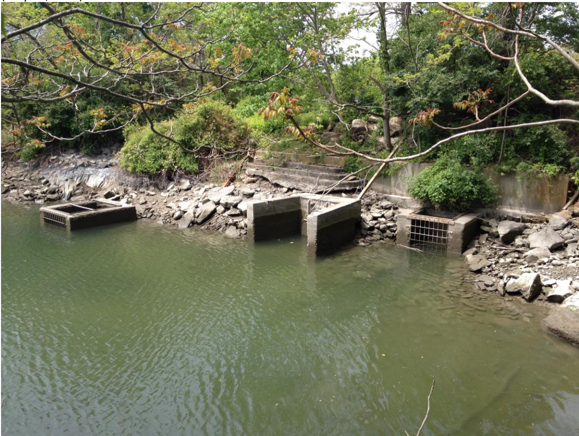
Photograph No. 8: Concrete control structures located along the shoreline of Delancey Cove. The control structures allow intermittent tidal flow to Golf Course Drainage System 3 (May 18, 2016).
