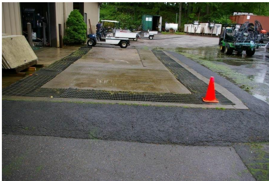
Figure 10-14. A retrofitted RGF system solid separation pad. Source: Robert Alonzi.
