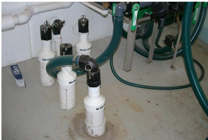
Figure 10-5. Recovery lines and trans pump in the equipment mixing and loading area. Source: Robert Alonzi.
