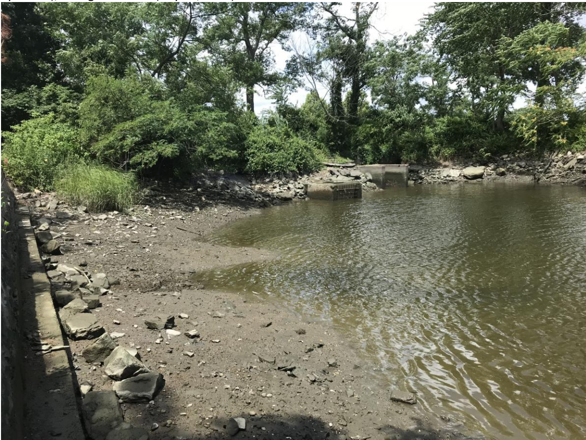
Photograph No. 7: View of tide gate openings along the northern shoreline of Delancey Cove, facing north (July 24, 2018). The tide gates regulate flow through culverts connecting Delancey Cove to Pond 10.
