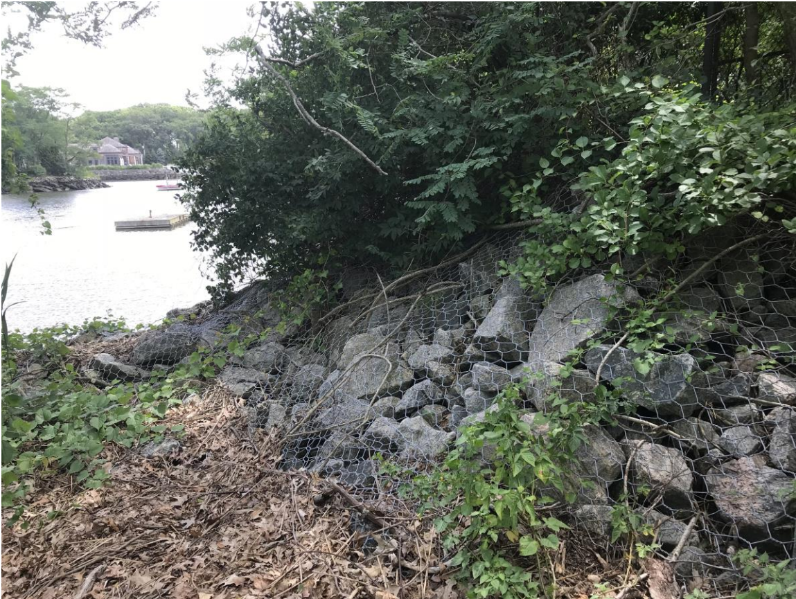
Photograph No. 4: View of rip-rap gabions along the Delancey Cove shoreline (July 31, 2018).
