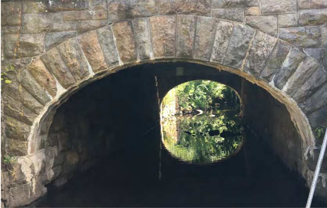
Figure 2-6: Close up of culvert end section (outlet).
