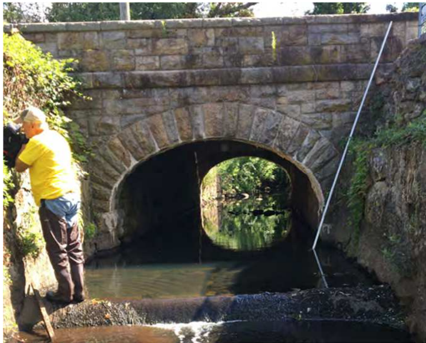
Figure 2-2: No culvert embankment due to retaining walls and parapet.
