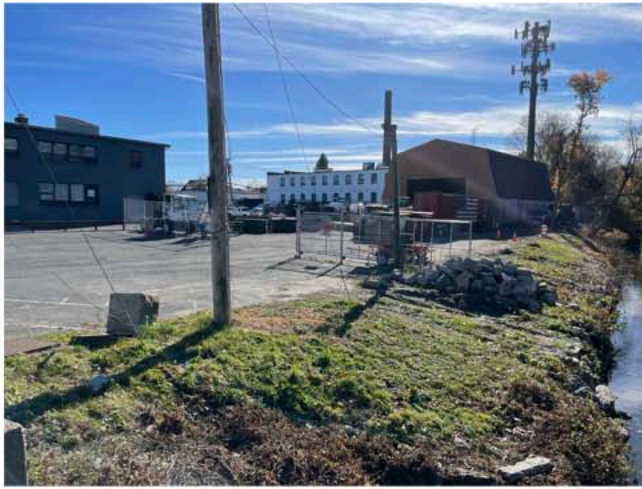
Village owned property containing a large salt shed is sited very close to the Sheldrake River.
