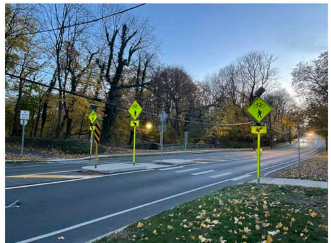
With Waverly Bridge under construction and the Center Ave. Pedestrian Bridge slated for demolition, Bub Walker Park is the only means for pedestrian access between the 2 neighborhoods separated by the river. A proper cross walk at this dangerous intersection is a necessity.
