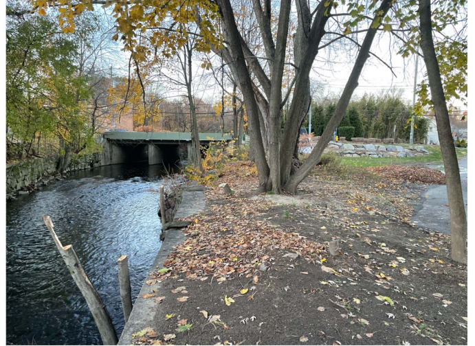
First Street Pocket Park looking north to the Barry Ave. Bridge.
