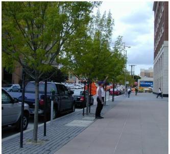
This installation uses cobble pavers with porous joints as the covering of a continuous trench of CU-Soil<sup>®</sup>.
