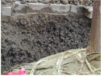
Closeup of CU-Structural Soil® after installation
