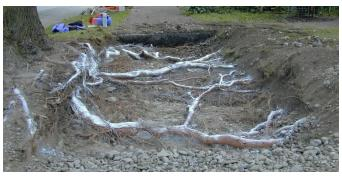
Thick superficial roots that have caused a sidewalk to heave.
