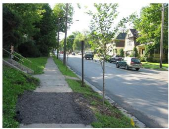
Because this tree lawn is so narrow, a sidewalk section has been removed, and a replacement will be poured on this CU- Soil® base. Ithaca, NY
