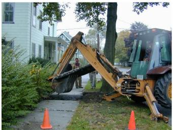
Removing this sidewalk section, and replacing it with one that has a CU- Soil<sup>®</sup> base, will allow tree roots to grow out from the tree lawn. Ithaca, NY
