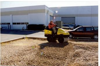
Installation and compaction of the CU- Soil<sup>®</sup>. Photo courtesy Southpine, Inc.
