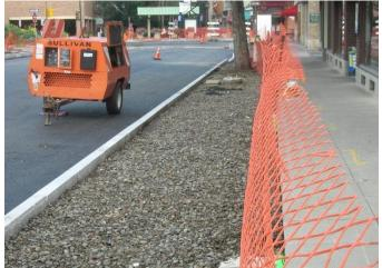
Installation of the new sidewalk on a base of CU-Soil®. This picture also shows an existing mature tree
