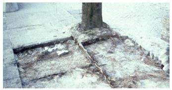
With paving removed, it is easy to see how this tree's roots took advantage of the weak points in the pavement. While the tree survived, the expanding roots caused the pavement to fail.
