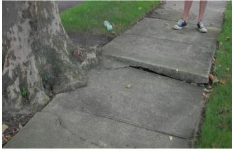
The roots of this tree have grown through the compacted soil beneath the sidewalk, into the large volume of soil beyond. Expanding tree roots have caused the sidewalk to heave.
