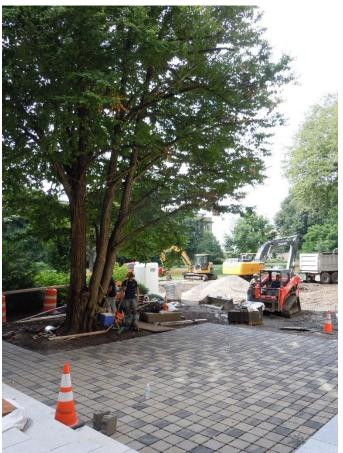
The roots of this katsura tree were threatened by construction of a new plaza. The tree was saved due to careful planning, and the use of CU-Structural Soil<sup>®</sup> around the existing tree roots. Pavers were installed directly on top of CU-Soil<sup>®</sup>
