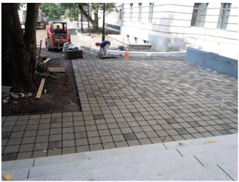
Permeable pavers were installed over the CU-Soil® and mature tree roots
