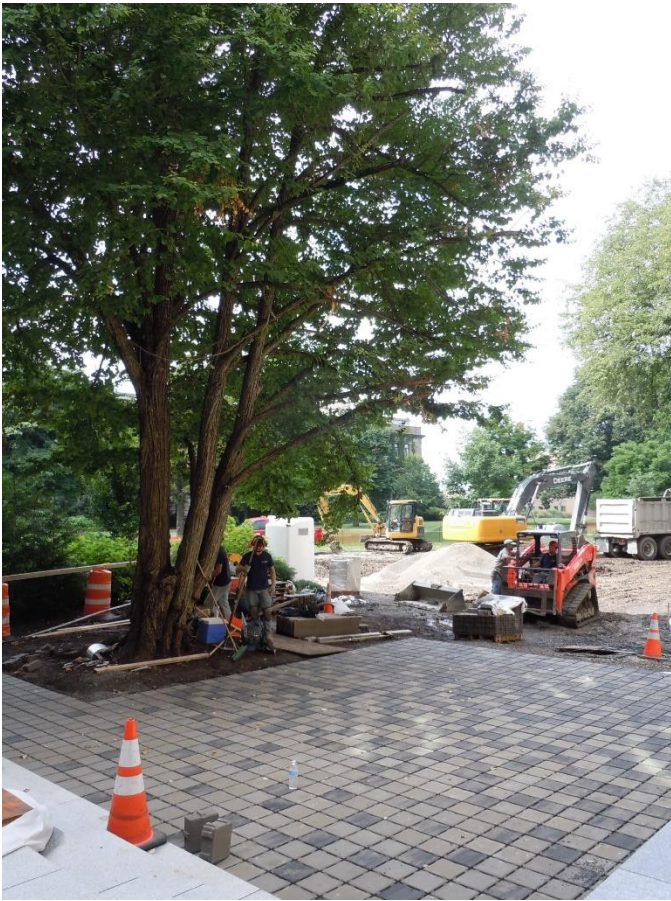
The nearly finished plaza space
