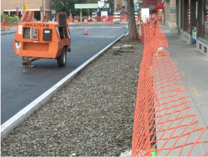
Renovation of this street and sidewalk in Ithaca, NY, provided an opportunity to use CU-Structural Soil® as a 36" base course for a replaced segment of sidewalk. This renovation allows the roots of this existing tree to escape its tree pit confines.
