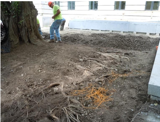
Soil around the roots was excavated using an air excavation tool
