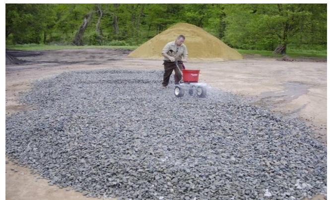
Gelscape® Tackifier being applied to uniformly sized crushed stone. Photo courtesy Amereq, Inc.
