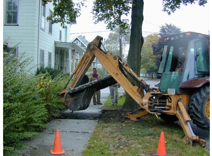
Removing this sidewalk section, and replacing it with one that has a CU- Soil® base, will allow tree roots to grow out from the tree lawn. Ithaca, NY
