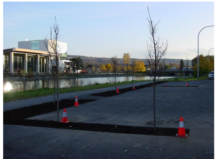
The finished parking lot
