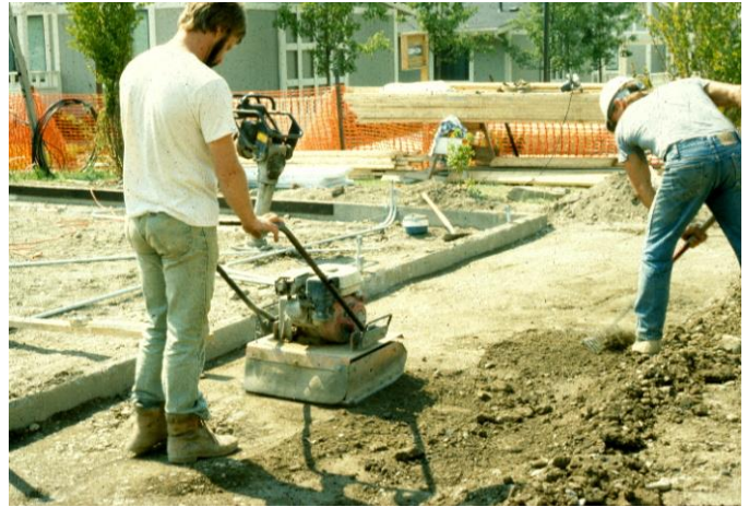
Compaction of soil in preparation for pavement
