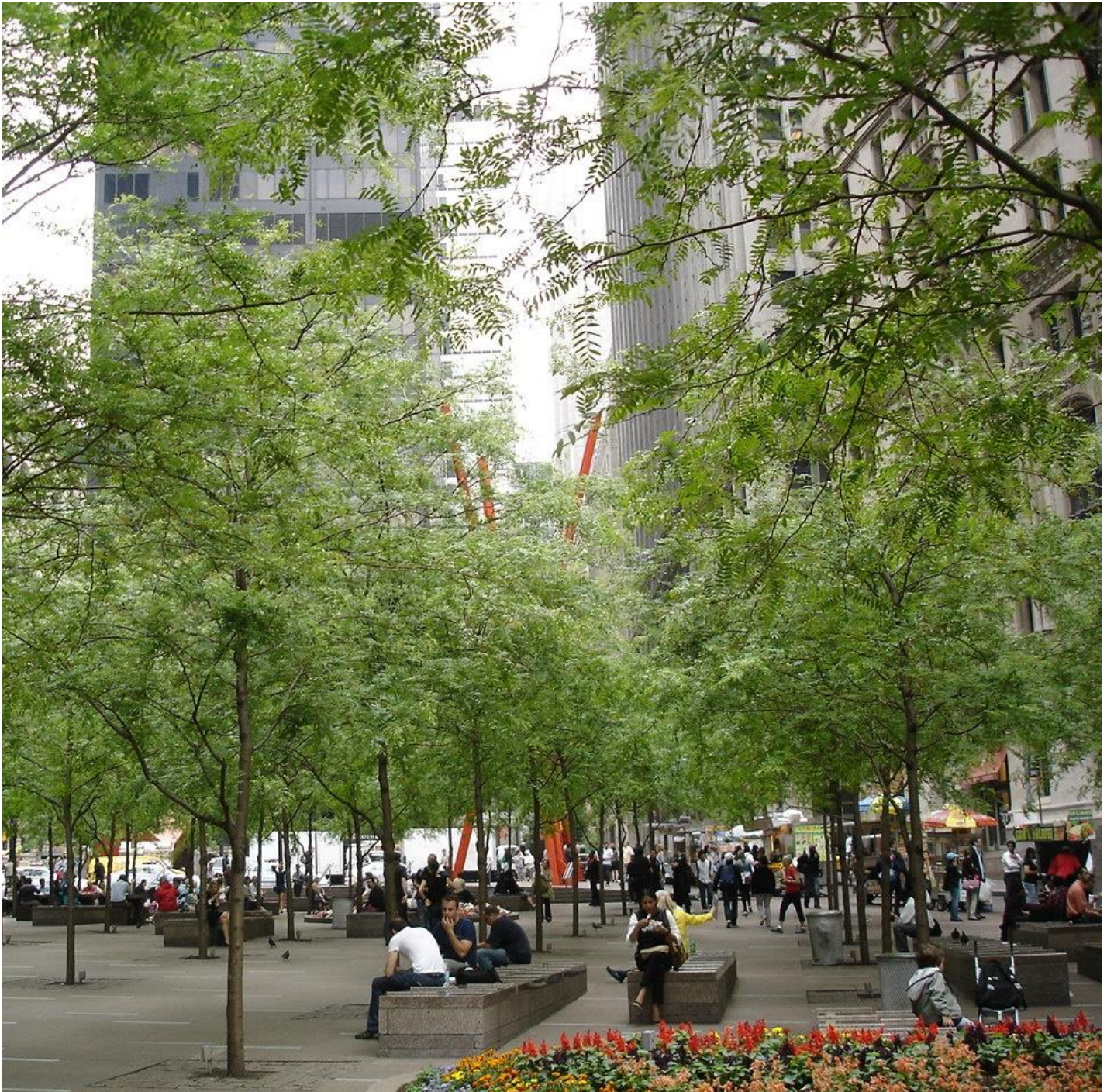
CU-Structural Soil® installation at Zuccotti Park, New York City
