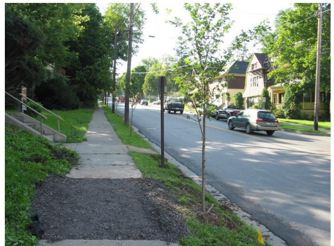
Because this tree lawn is so narrow, a sidewalk section has been removed, and a replacement will be poured on this CU- Soil® base. Ithaca, NY
