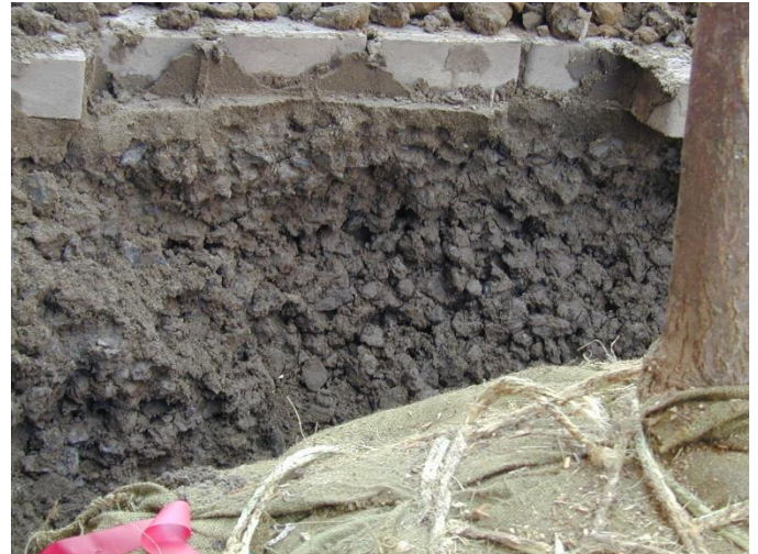
Closeup of CU-Structural Soil® after installation
