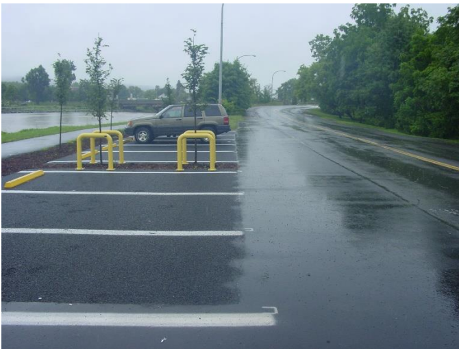
A porous asphalt and CU-Soil® installation in Ithaca, NY just after construction
