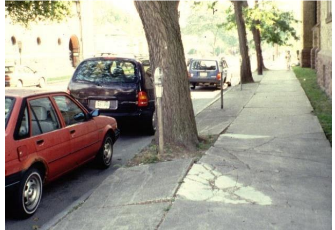
Trees planted in severely limited soil volumes die young unless their roots are able to break past compacted soils into an adequate volume of useable soil. This often results in dangerous sidewalk heaving.
