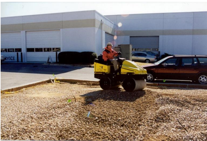
Installation and compaction of the CU- Soil®. Photo courtesy Southpine, Inc.
