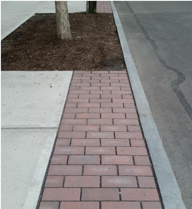
By having porous joints between the bricks in this paving strip, water is able to infiltrate into the CU-Soil® below. Ithaca, NY.
