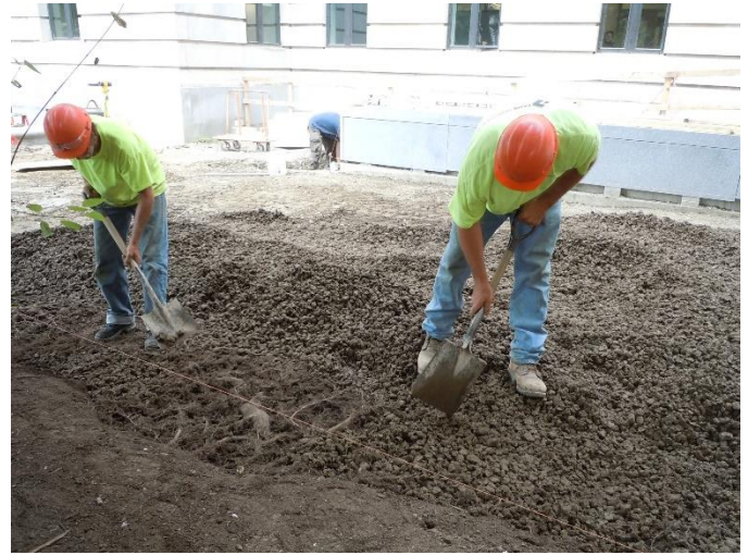
12"-15" of CU-Soil® was placed on top of the exposed roots and compacted for use as a base course for the paving
