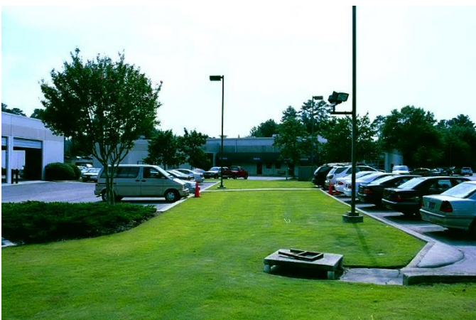
The finished installation. Photo courtesy Southpine, Inc.
