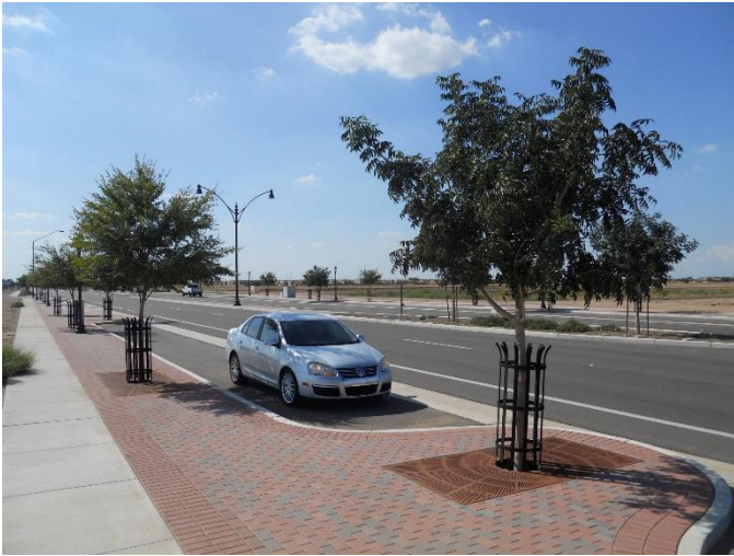
This new streetscape in Phoenix, Arizona provided an opportunity to incorporate a large volume of CU-Structural Soil® beneath the pavers. Photo courtesy AZ Best, LLC
