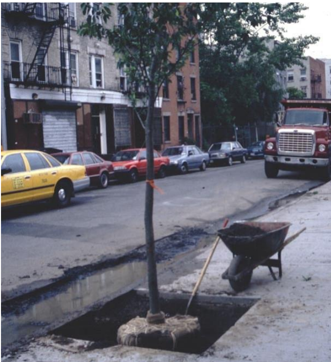
The standard (but entirely inadequate) city tree pit. It's not surprising that trees in these situations have shorter lifespans.
