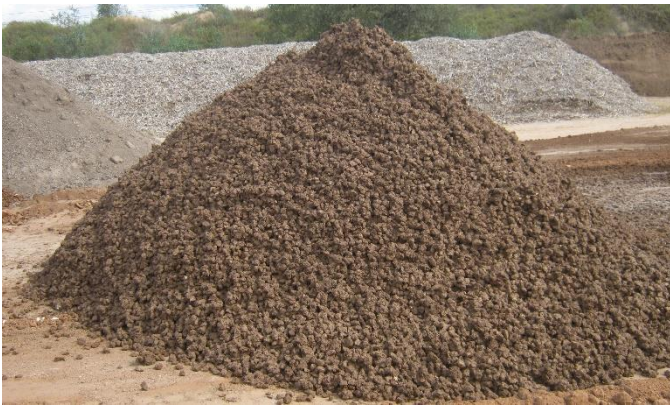
Clay loam soil is mixed with the crushed stone. The added Gelscape® Tackifier helps it “stick” and prevents settling during construction. Photo courtesy J-V Environmental Services
