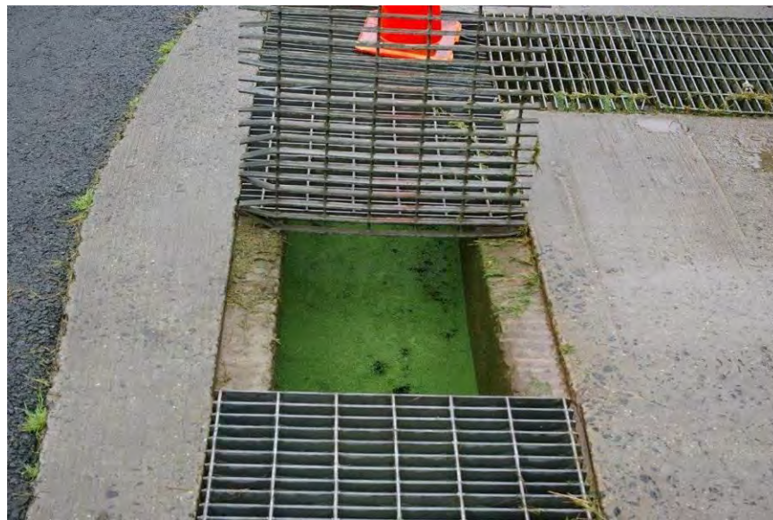
Figure 10-13. A Retrofitted RGF system separates solids in the wash water. Source: Robert Alonzi.
