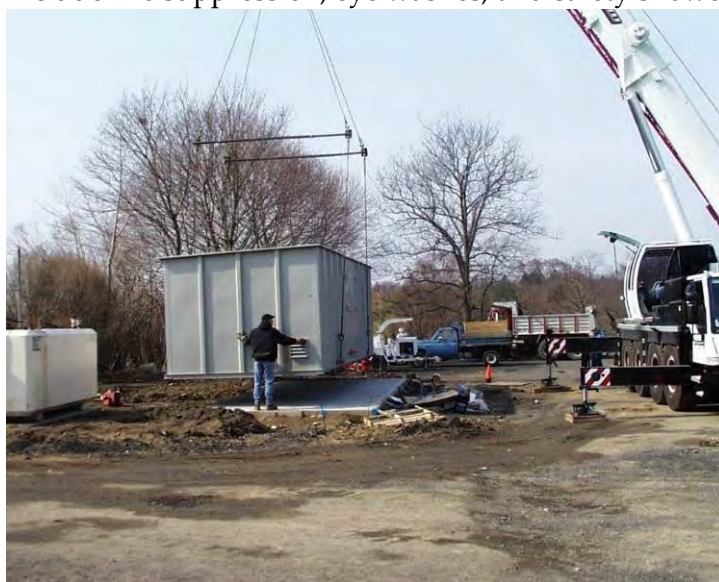
Figure 10-2. Modular containment units can be installed in many sizes. Source: Robert Alonzi.
