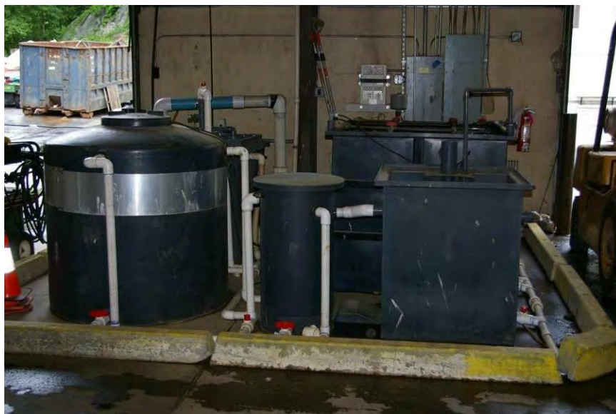
Figure 10-9. Microbial system for treating wastewater. Source: Robert Alonzi.
