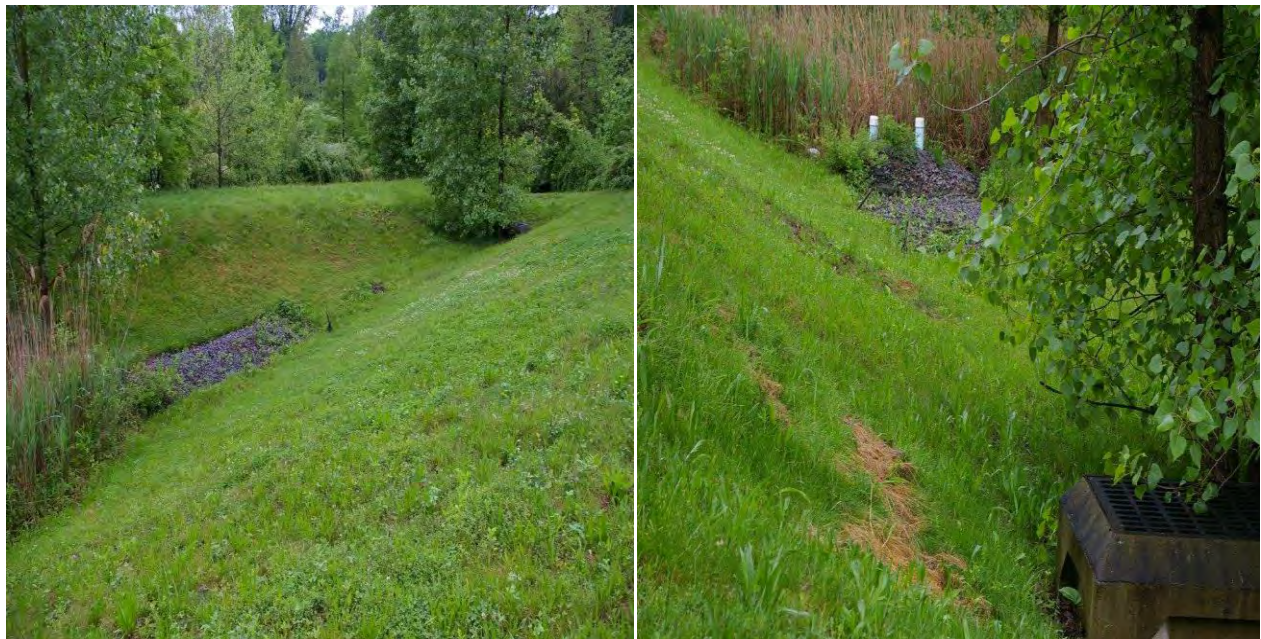
Figure 4-1. Grasses filter strips discharging into water filtration basins. Source: Robert Alonzi.
