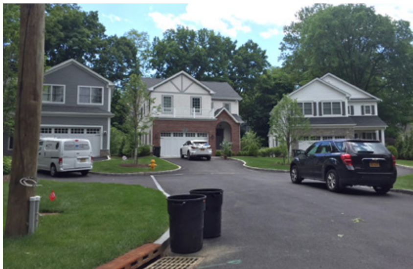
Figure 70: A new subdivision in the Village that resulted in three new houses.
