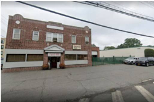
Figure 95: A wide expanse of asphalt fronts this building along Mamaroneck Avenue
