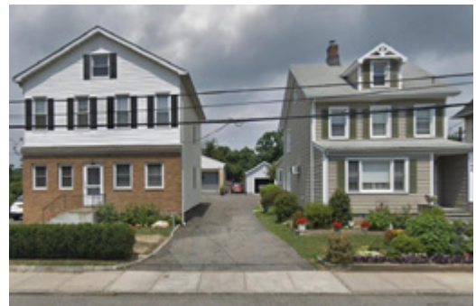
Figure 99: Houses located on Halstead Avenue
