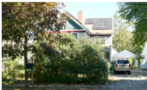
Figure 61: A house in the Village with rooftop solar panels.
