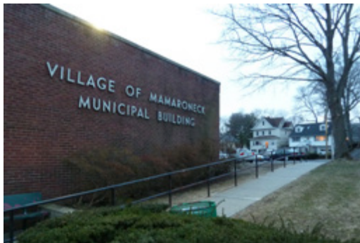
Figure 149: The Municipal Building at 123 Mamaroneck Ave
