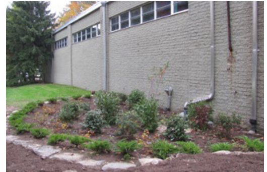
Figure 139: A rain garden collects runoff from the downspout of a municipal building (photo by Town of Mt. Pleasant)
