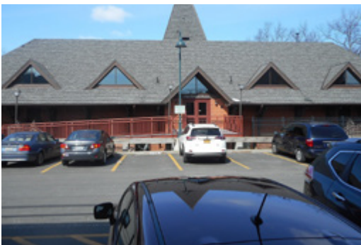
Figure 5: The train station parking lot is at capacity, and there is a long waiting list. Parked among commuter vehicles in the lots are two ZipCars
