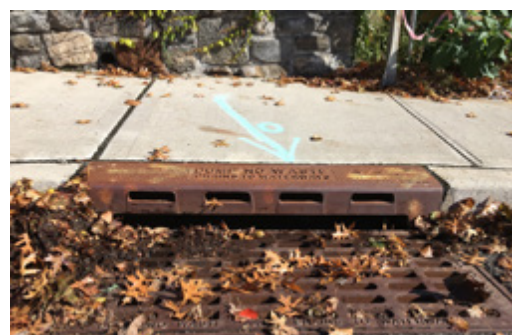
Figure 38: A newly-installed catch basin in the Village.
