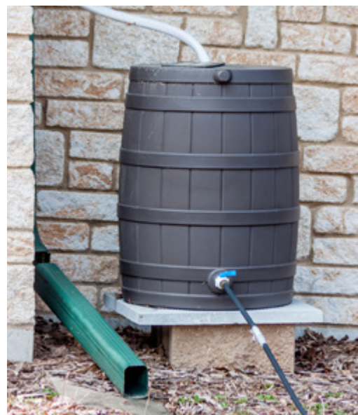
Figure 40: A rain barrel collects water from a roof of a house, which reduces stormwater runoff.
