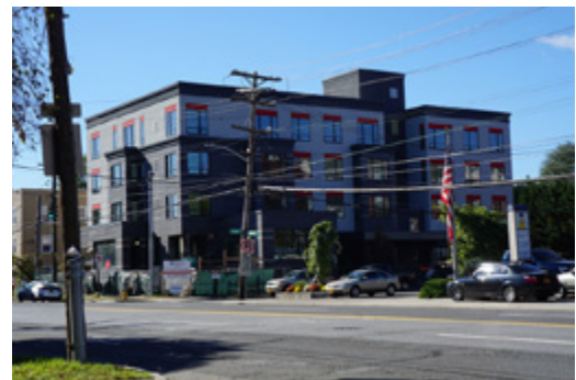
Figure 3: A newly-constructed building in the Village’s transit-oriented development overlay zone.
