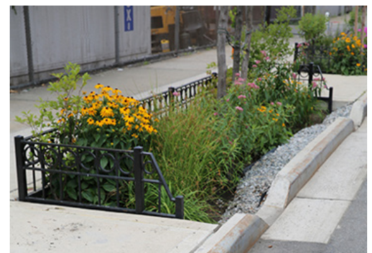
Figure 58: A bioswale, a type of green stormwater management technique, is designed to collect and absorb stormwater from the street before it enters the sewer system.
