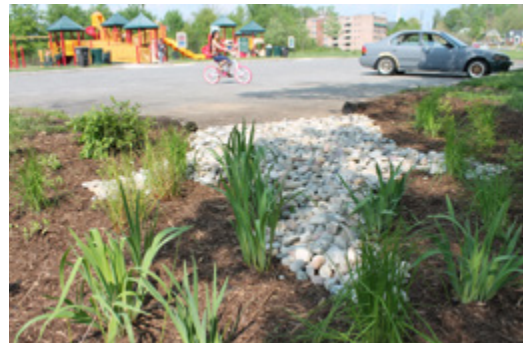
Figure 140: A rain garden collects runoff from a playground parking lot (photo by Elvert Barnes, licensed by CC BY-SA 2.0)
