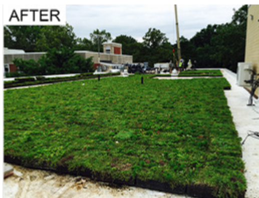
Figure 55: Before and after images of the Sarah Neuman Center’s green roof.
