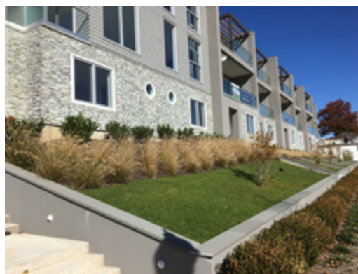
Figure 41: A new townhouse development along Post Road West utilizes green infrastructure, or vegetation to filter and absorb stormwater runoff.
