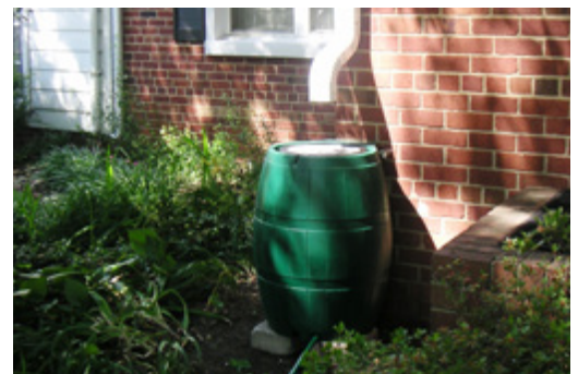
Figure 141: A rain barrel collects rainwater from the roof of a home (photo by Arlington County, VA)
