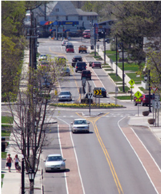
Figure 118: Route 62 in Hamburg, NY was redesigned through a Complete Streets approach (photo by NYSDOT)
