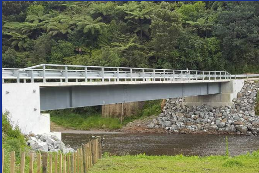
Traditional Steel Girders
