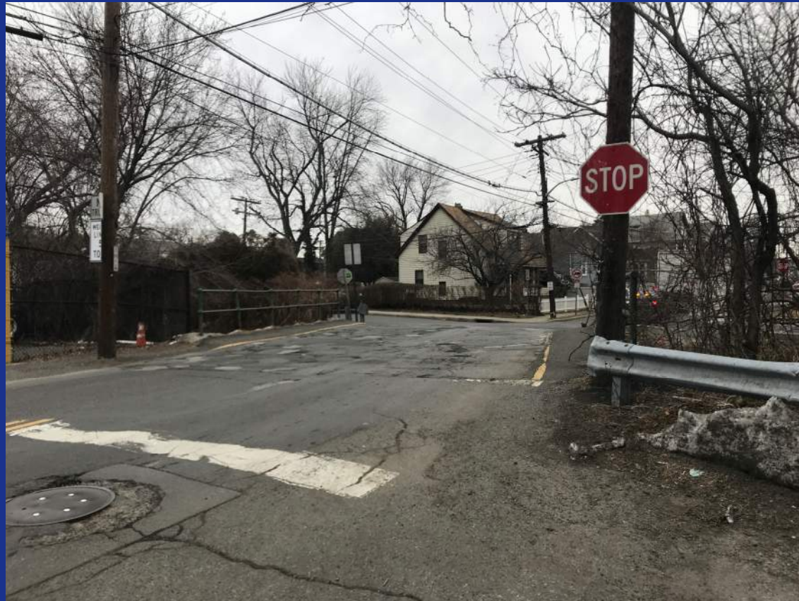
Bridge Deck (Looking North)
