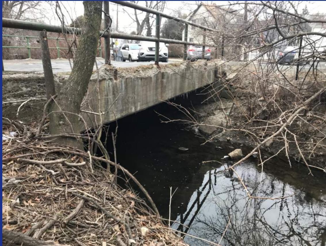
Southeast Bridge Fascia
