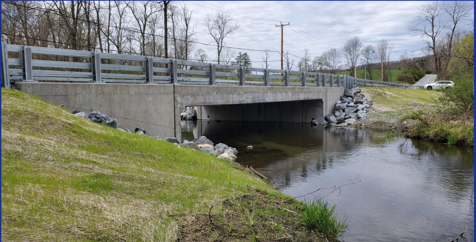
Three-Sided Precast Concrete Structure
