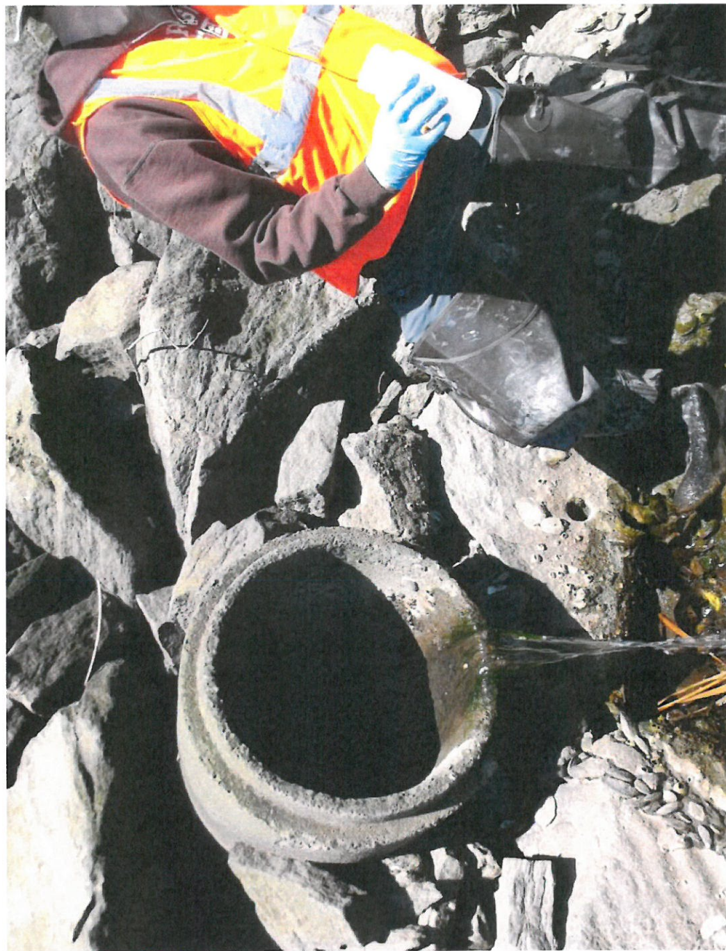
VJ-58, Flow measured 2.6 gpm, algae and light bacteria growth. Outfall from Lawn Terrace.
