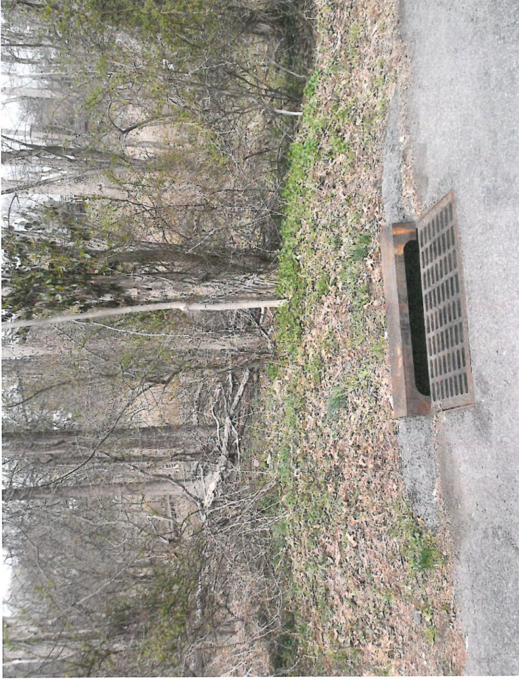
VJ-65 catch basin. Dye tested, but could not confirm connection to outfall (not pictured).
