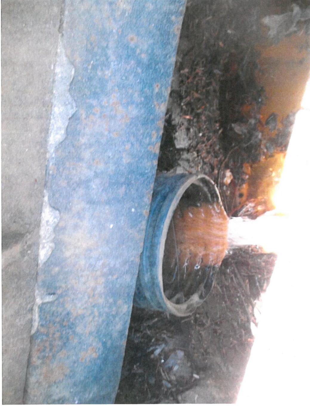
Sampling point for VJ-54a. Bacteria growth present.
