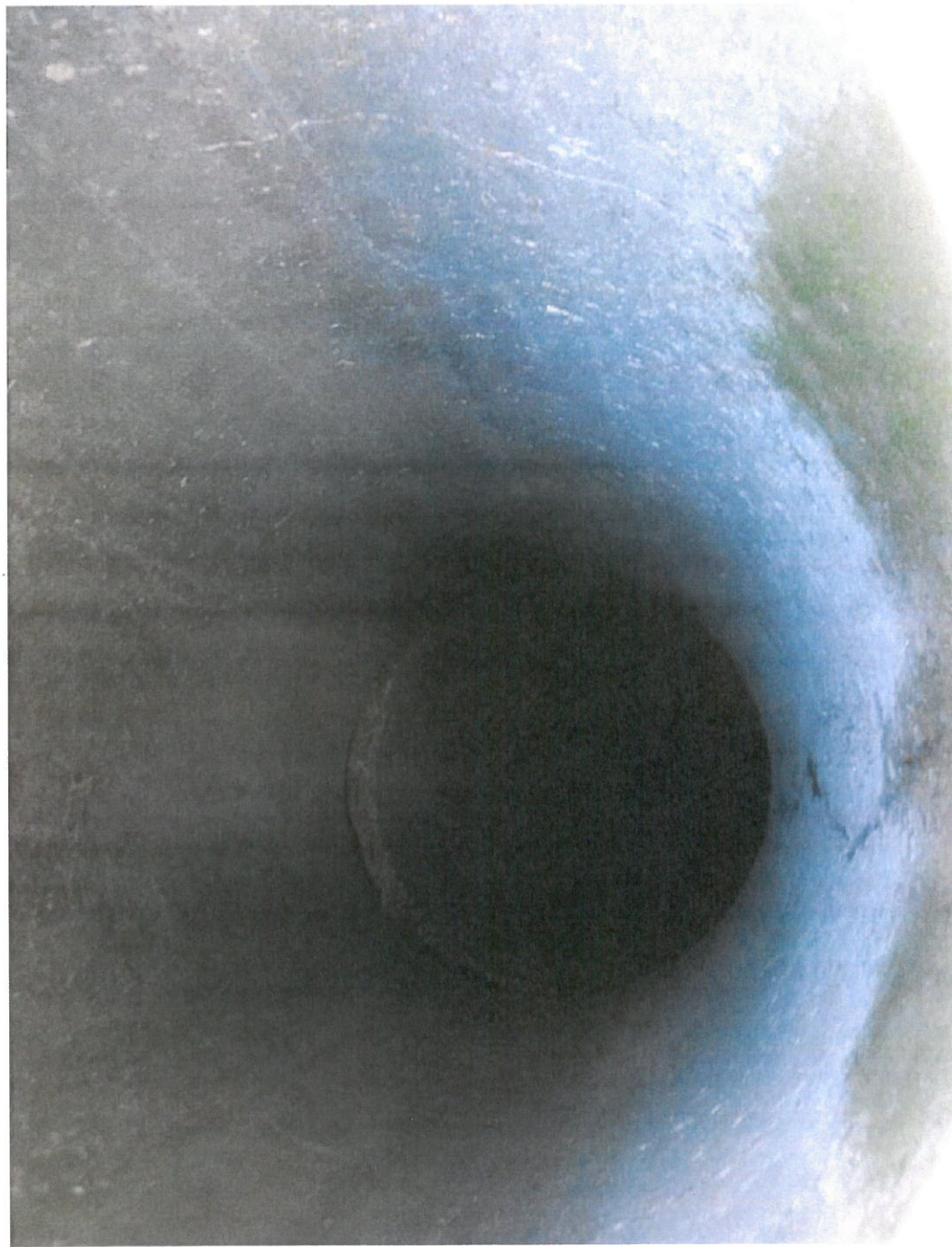
VJ-54a interior. Pipe is separated 7ft. in from outfall, allowing flow into retaining wall.
