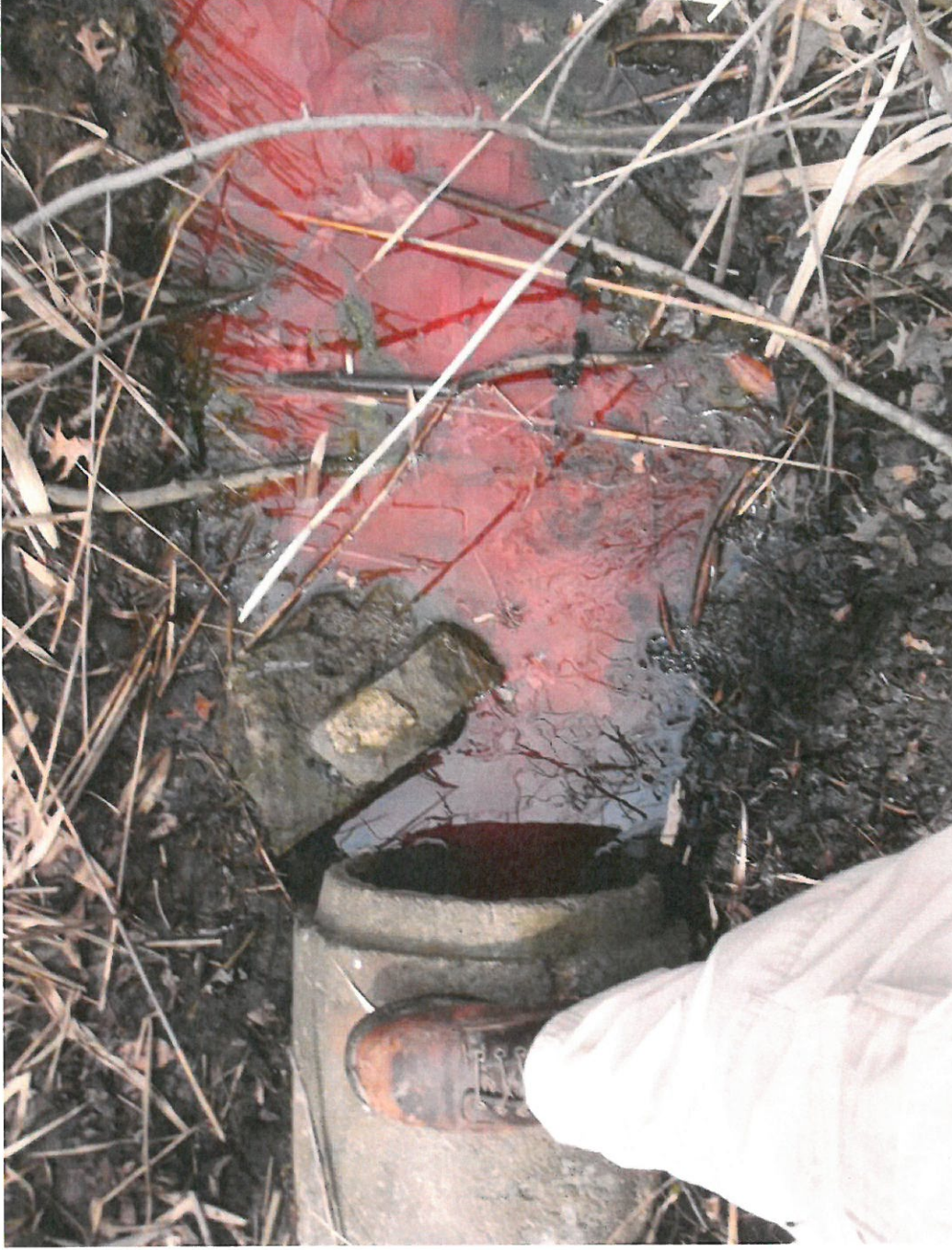
VJ-61 dye tested to confirm US CB.
