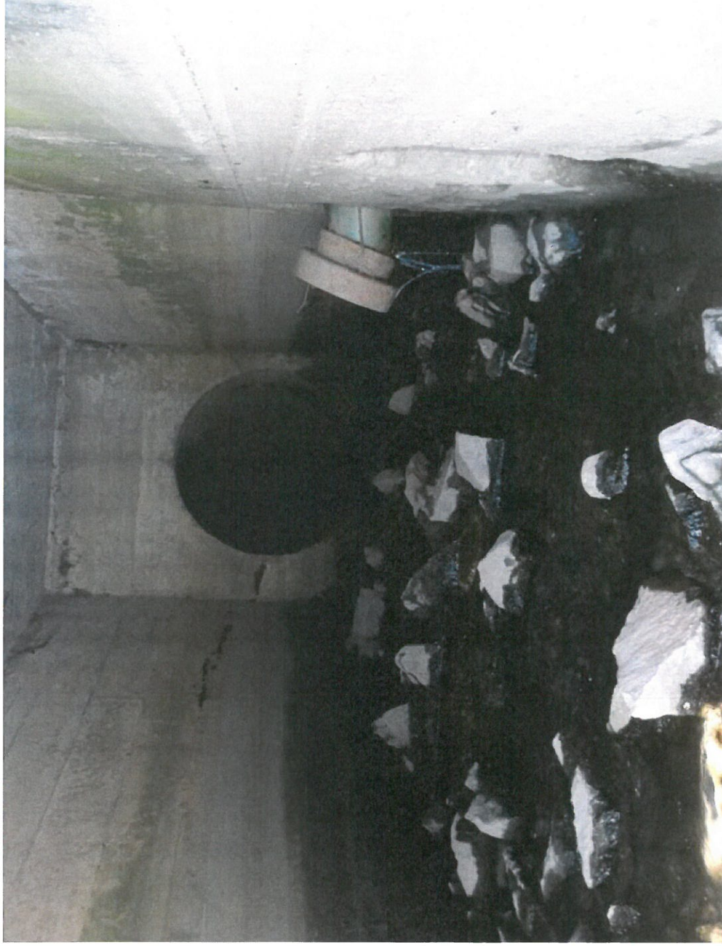
VJ-04 interior. Two additional inlets at 3 o'clock.
