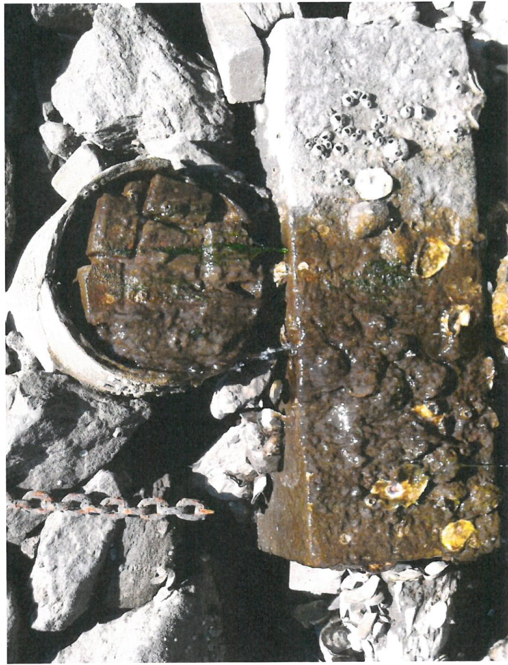
BSB-29, Flow measured at 0.36 gpm, maybe more from cracks in pipe. Outfall from Lawn Terrace.
