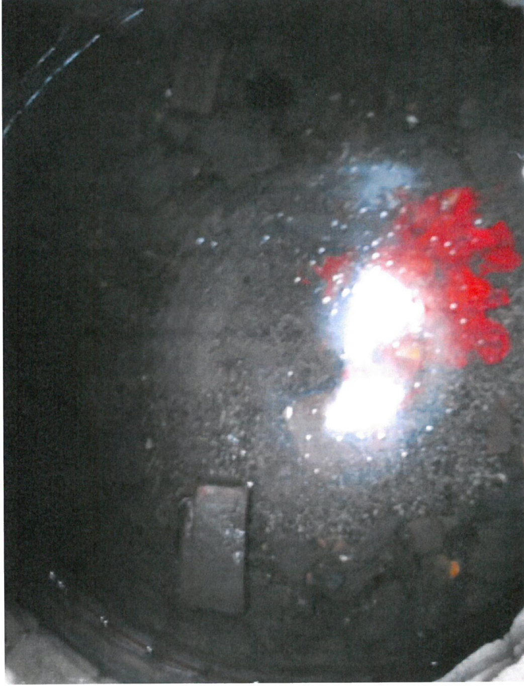
USMH_VC-18 interior. No flow into MH, dye tested pool of water. No outgoing flow.
