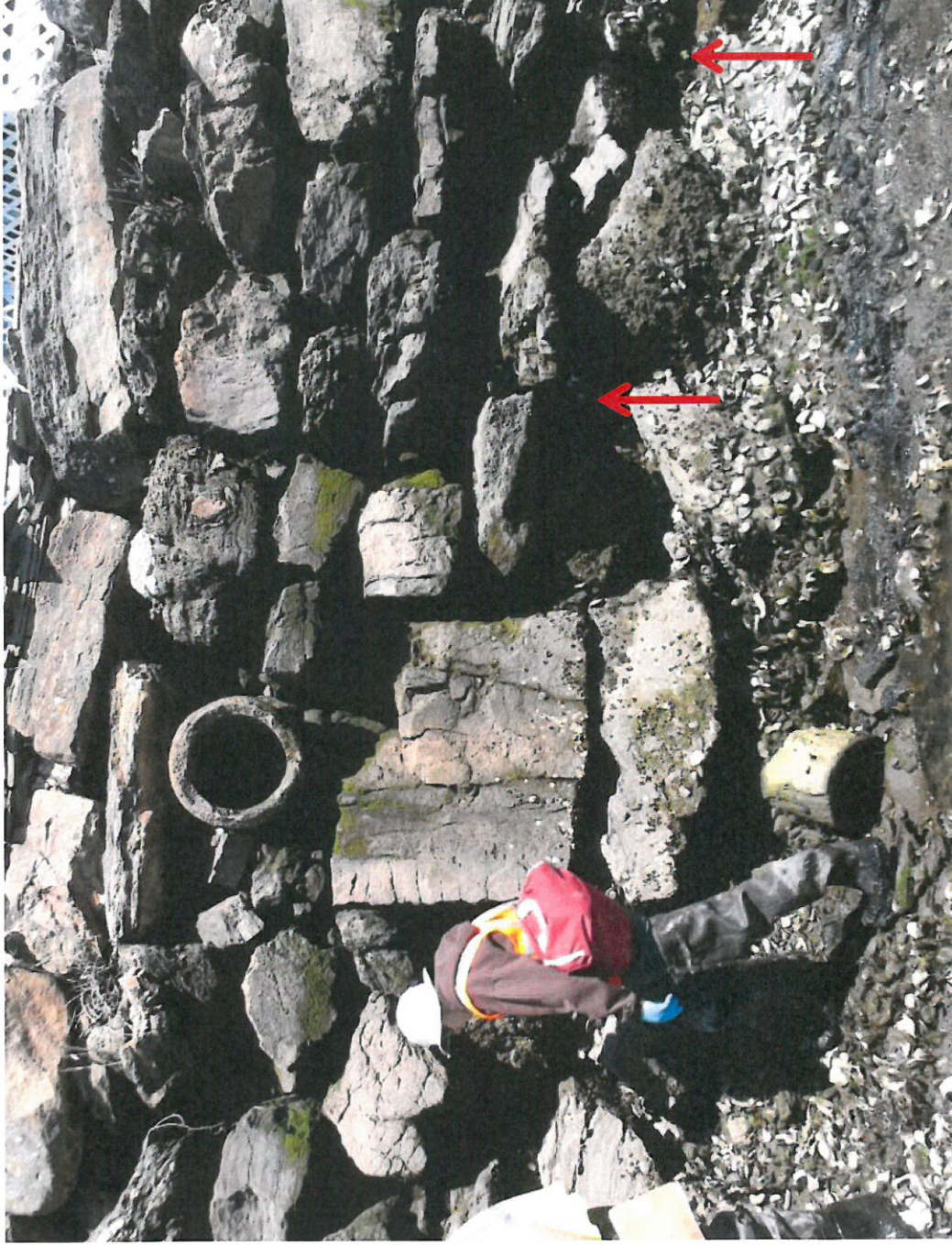
VJ-54a Outfall exterior at low tide. Flow visible through retaining wall face. Outfall from Guion Dr and Lawn Terrace intersection.
