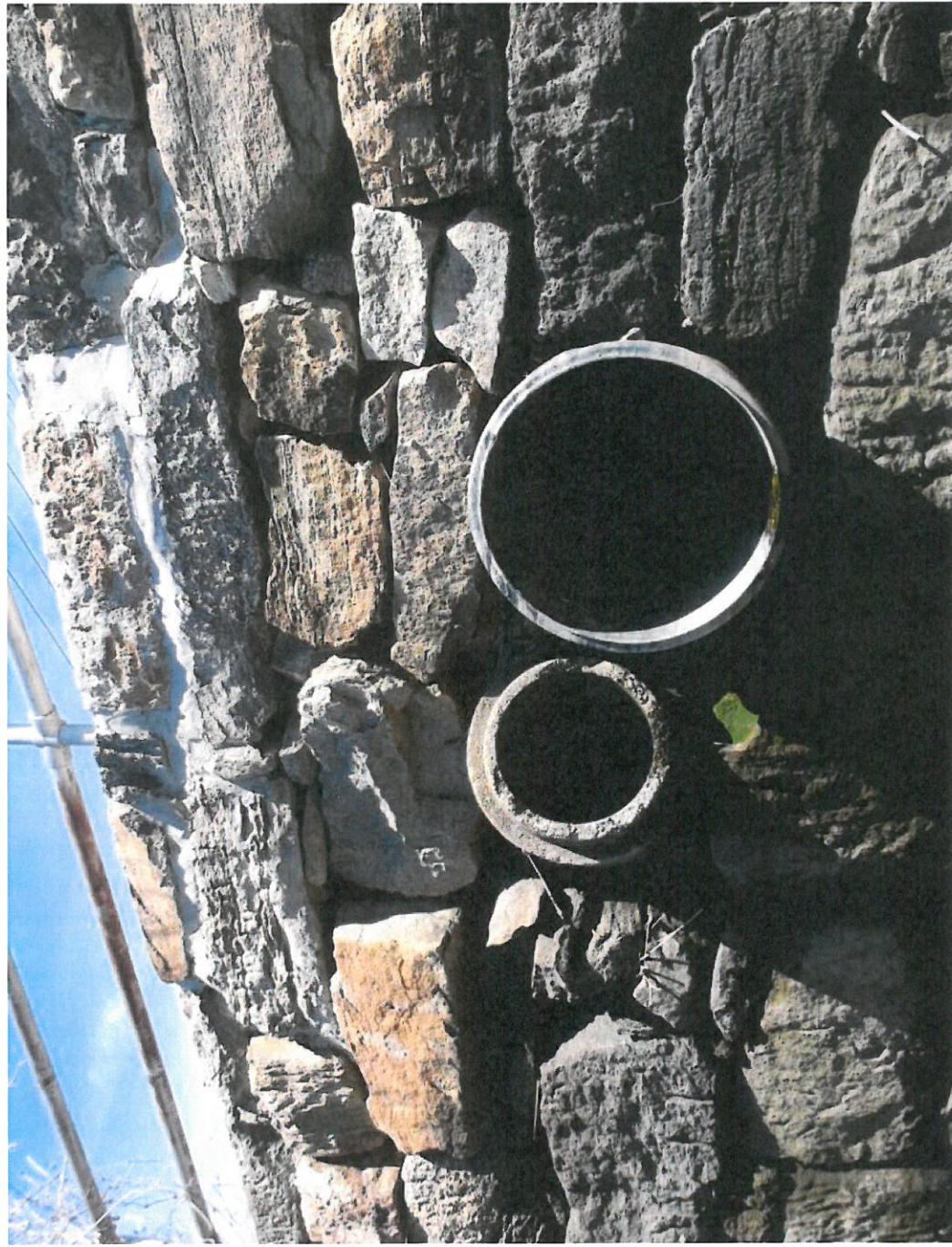
VJ-57 wet pipes and wall face. Very slow dripping. Outfall from S Barry Ave at bridge.
