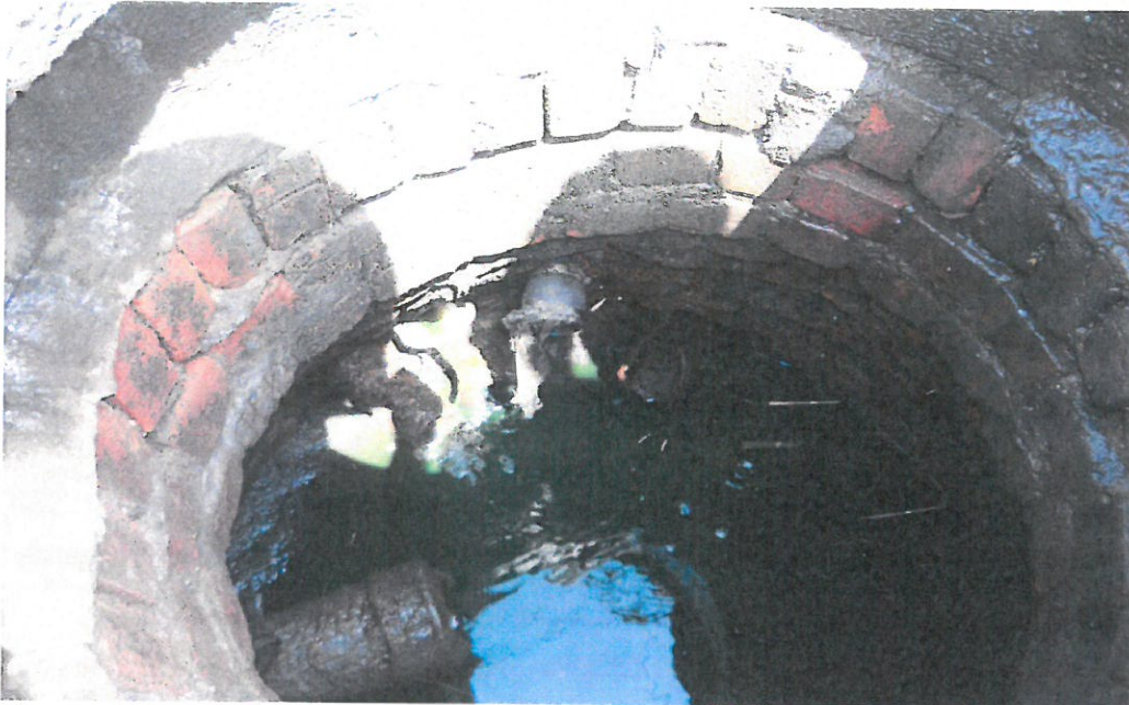
Photo #6: Sanitary sewer manhole in front of Village DPW Garage – Green dye from dye test of curtain drains at north end of Fayette Avenue and DPW Garage floor drains. Incoming pipes from Village DPW Garage floor drains and the transfer station pump station shown at the top of the photo.
