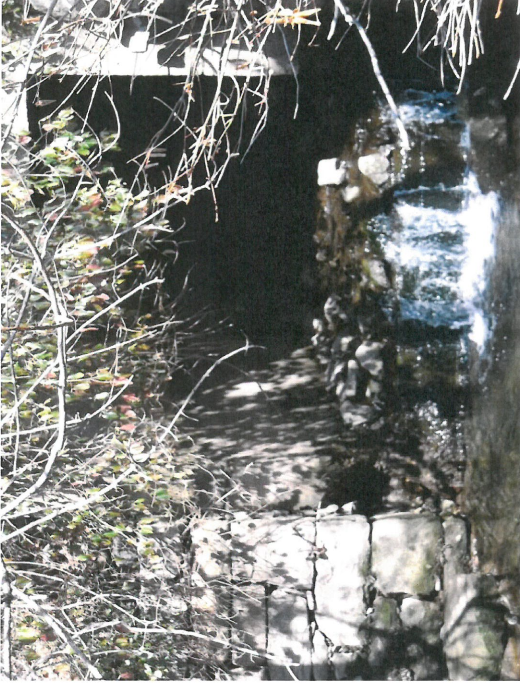
Outfall VJ-04. Flow rate 93 gpm. Light odor and some algae growth.
