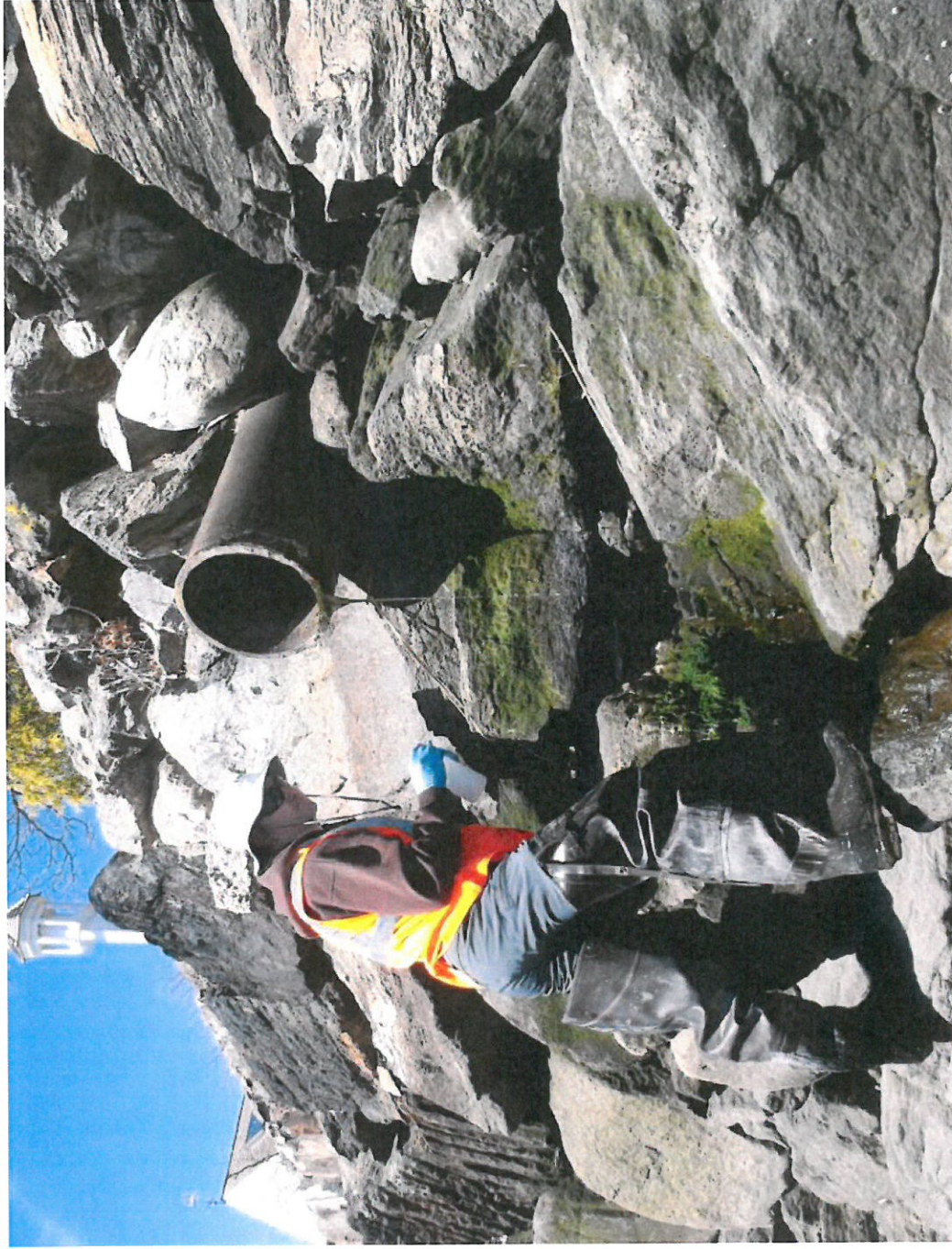
BSB-28, Flow rate 0.1 gpm. Algae growth present. Outfall from Lawn Terrace.
