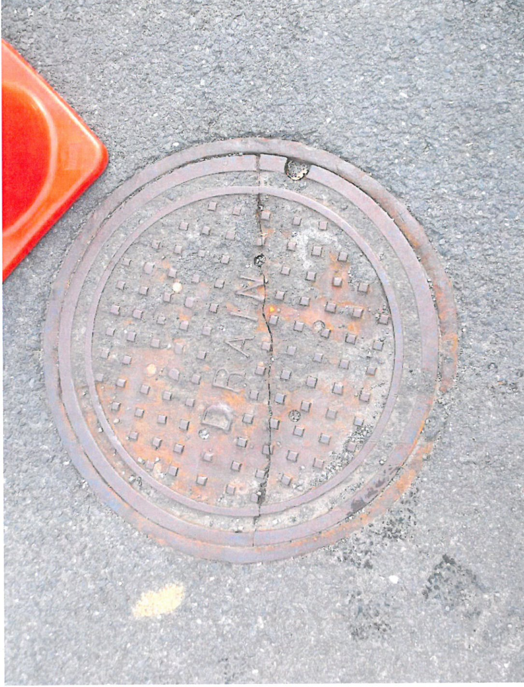
USMH_VC-18, exterior. Lid cracked in half.
