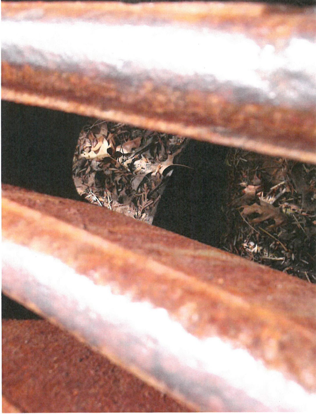
BSB-24 upstream catchment basin. Dry with metal cap over outlet. Filled with leaves and debris.
