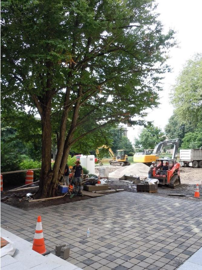
*The roots of this katsura tree were threatened by construction of a new plaza. The tree was saved due to careful planning, and the use of CU-Structural Soil® around the existing tree roots. Pavers were installed directly on top of CU-Soil®*
