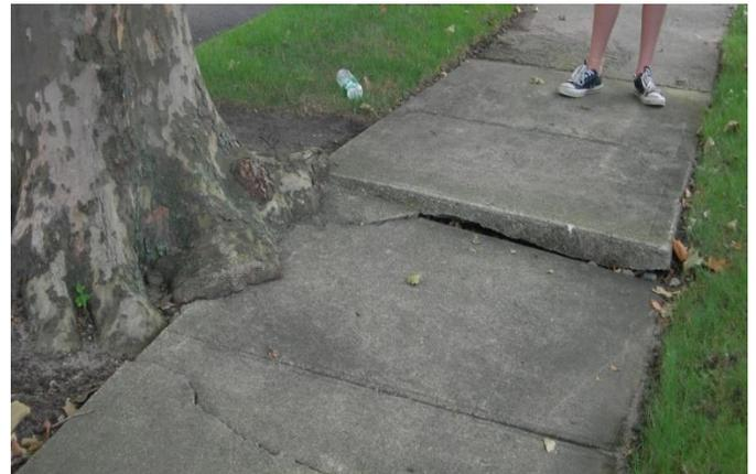
*The roots of this tree have grown through the compacted soil beneath the sidewalk, into the large volume of soil beyond. Expanding tree roots have caused the sidewalk to heave.*
