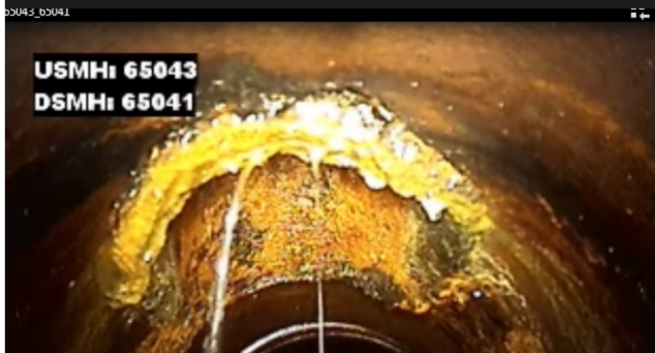
Infiltration and Mineral Deposits
