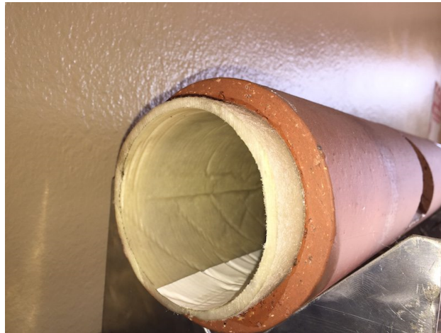
Clay Pipe With Liner
